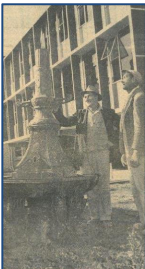
Installation of Fountain at Trustees Court
